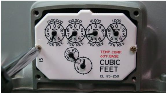
4. Set the index aside where it will not be damaged or fill with dirt, rain or snow. The index will be mounted in the endpoint later in this procedure. Verify the index mounting screws are 5/8" long and not corroded. If the screws are the correct length and not corroded, retain for later use. If the original screws are discarded, use the correct replacement screws (see [Installation Prerequisites](#) on page 7.)
