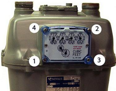
2. Examine the mounting screws. If they are 5/8" long and not corroded, keep them to attach the 100G Datalogging gas endpoint assembly. If the screws are not the correct length or if the screws are corroded, discard.
