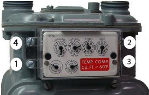
2. Examine the mounting screws. If they are 5/8" long and not corroded, keep them to re-attach the 100G Datalogging gas endpoint assembly. If the screws are not the correct length or if the screws are corroded, discard.
